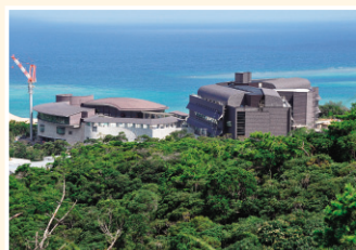
The Center Building (left) and Laboratory 1
